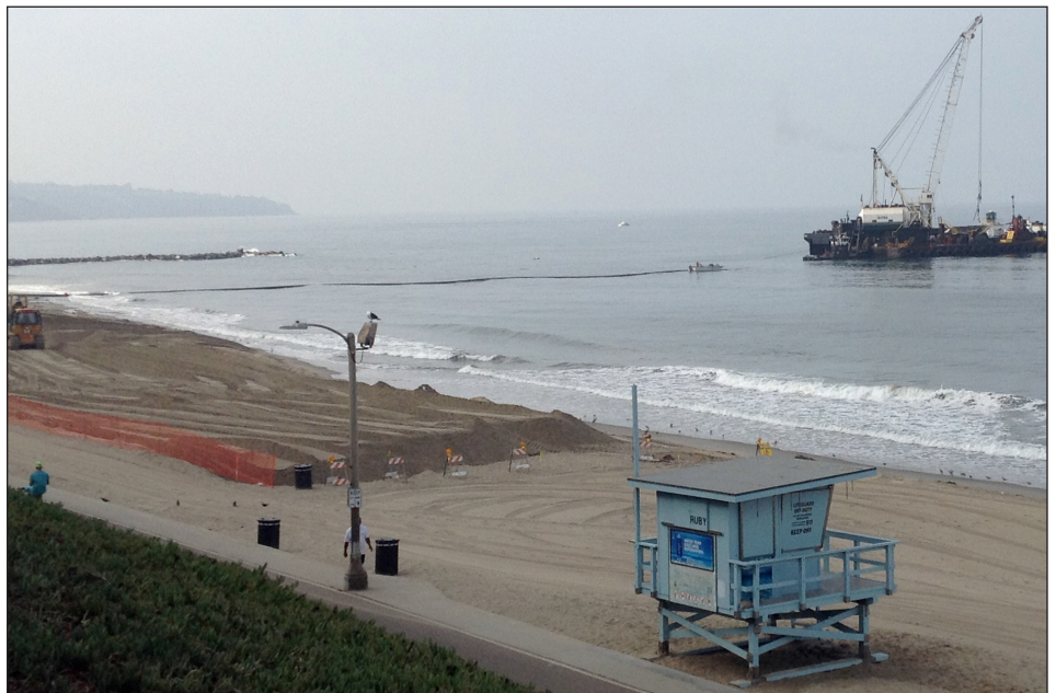
Dutra Dredging Company puts the final touches on the placement of nearly 75,000 cubic yards of sand at Redondo Beach as part of the Marina del Rey entrance channel navigation project shortly before the dredge Paula Lee departed and bulldozers contoured the sand to meet the required beach profiles. (USACE photo by Greg Fuderer)
