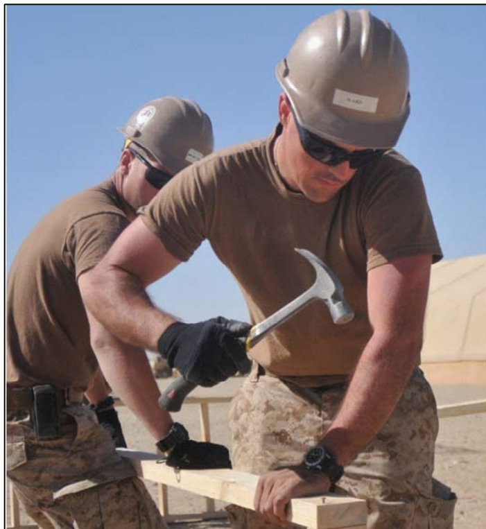
photo by Mass Communication Spec. 1st Class Steven Myers Warner Ward, a member of Naval Mobile Construction Battalion 133's Echo Company, drives the first nail of a new base form during the construction of a K-span building project.
