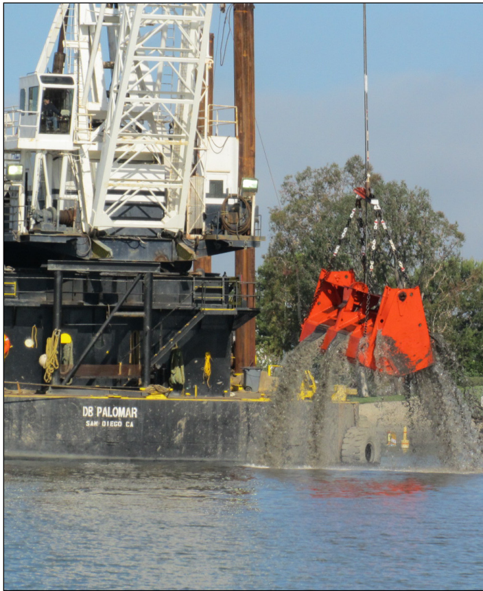
R.E. Staite's dredge Palomar works in tight spaces alongside waterfront homes in Newport Harbor to remove sediment from channels, restoring safe navigation for boats using the harbor. (Photo courtesy of Chris Miller, Newport Beach Harbor Resources Manager)
