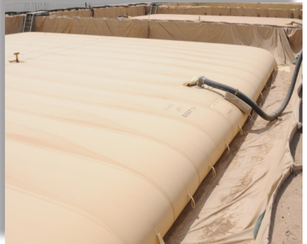
CAMP ARIFJAN, Kuwait - When full, this fuel bladder, nestled in a berm of earth, will provide fuel for military and civilian contacted vehicles conducting logistic and sustainment operations throughout Kuwait. (U.S. Army photo by Sgt 1st Class Keith Warzon, 113th Sustainment Brigade Public Affairs).
