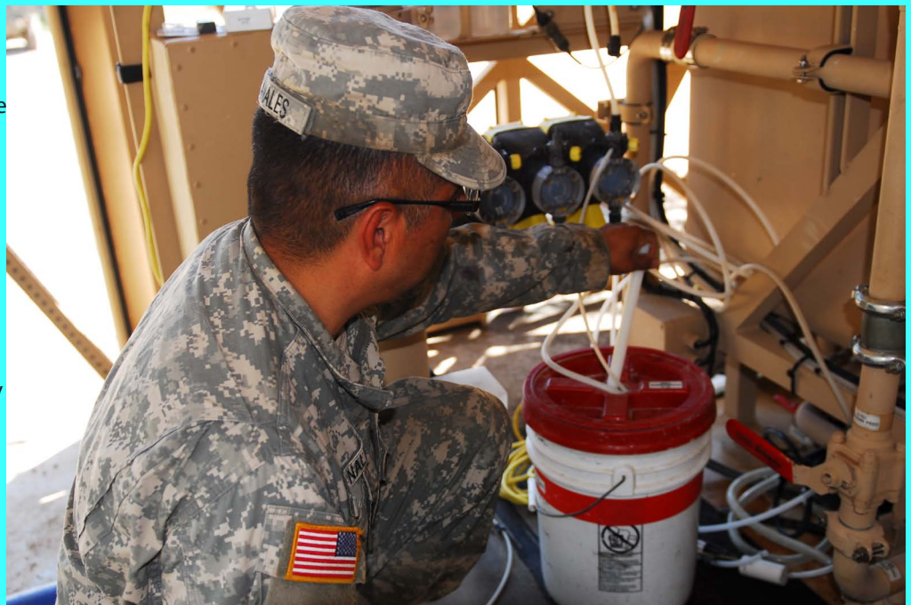
Spc. Reynaldo Canalas, checks the chlorine mixture of the Tactical Water Purification System) as part of the required hourly tests he performs as the 288th Quartermaster Detachment provides clean water in support of the Combat Support Training Exercise 91 12-01.
