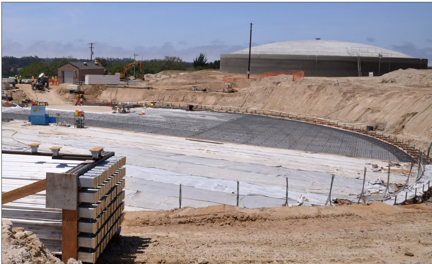
Corps contractors construct the second of two new 4-million-gallon water reservoirs May 11 at Vandenberg AFB, Calif. The new water tanks support a population of more than 18,000 military, family members, contractors and civilian employees at the base. (USACE photo by Dave Palmer)
