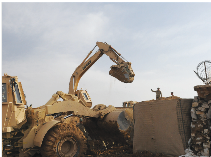
Soldiers with 1022nd Vertical Engineer Company, 578th Engineer Battalion, use an excavator to fill Hesco barriers to secure the perimeter on Forward Operating Base Arian March 14. The Louisiana National Guard unit has completed several building projects on FOB Arian as part of Operation Devil Hammer. (Photo by U.S. Army Staff Sgt. Catrina Dorsey, RC-East PAO)
