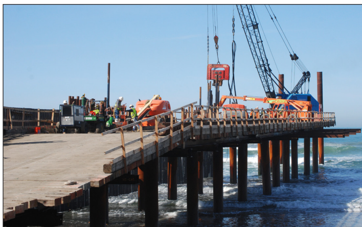
The temporary pier enabled the contractor to overcome obstacles unique to working in a surf zone. (USACE photo by Greg Fuderer)
