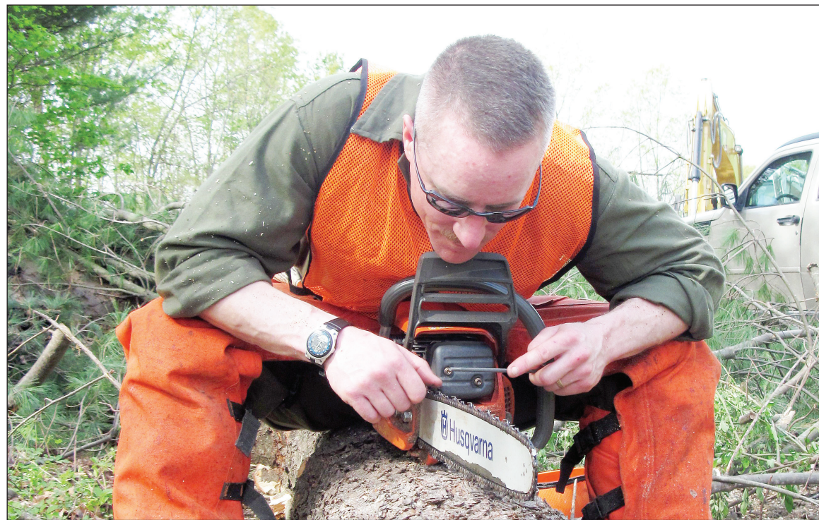
Air Force Master Sgt. Gerald Hedstrom, 477th Civil Engineer Squadron, sharpens a chain saw during construction of the Boy Scout Jamboree site. (Photo by Air Force Master Sgt. Brede Emtman)
