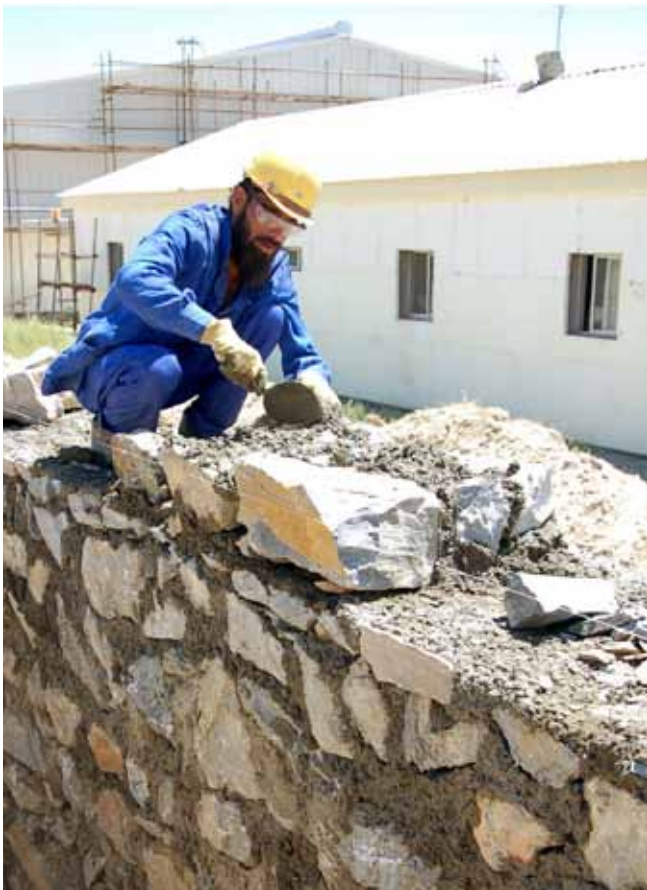
This skilled Afghan wall builder is one of between 500 to 650 workers who are providing for their families every day at Camp Morehead.
