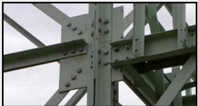
Close-up view demonstrating how the steel angle bars are assembled and bolted together.
