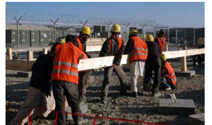
Afghan workers installing supports into place. (Photo by David Salazar)
