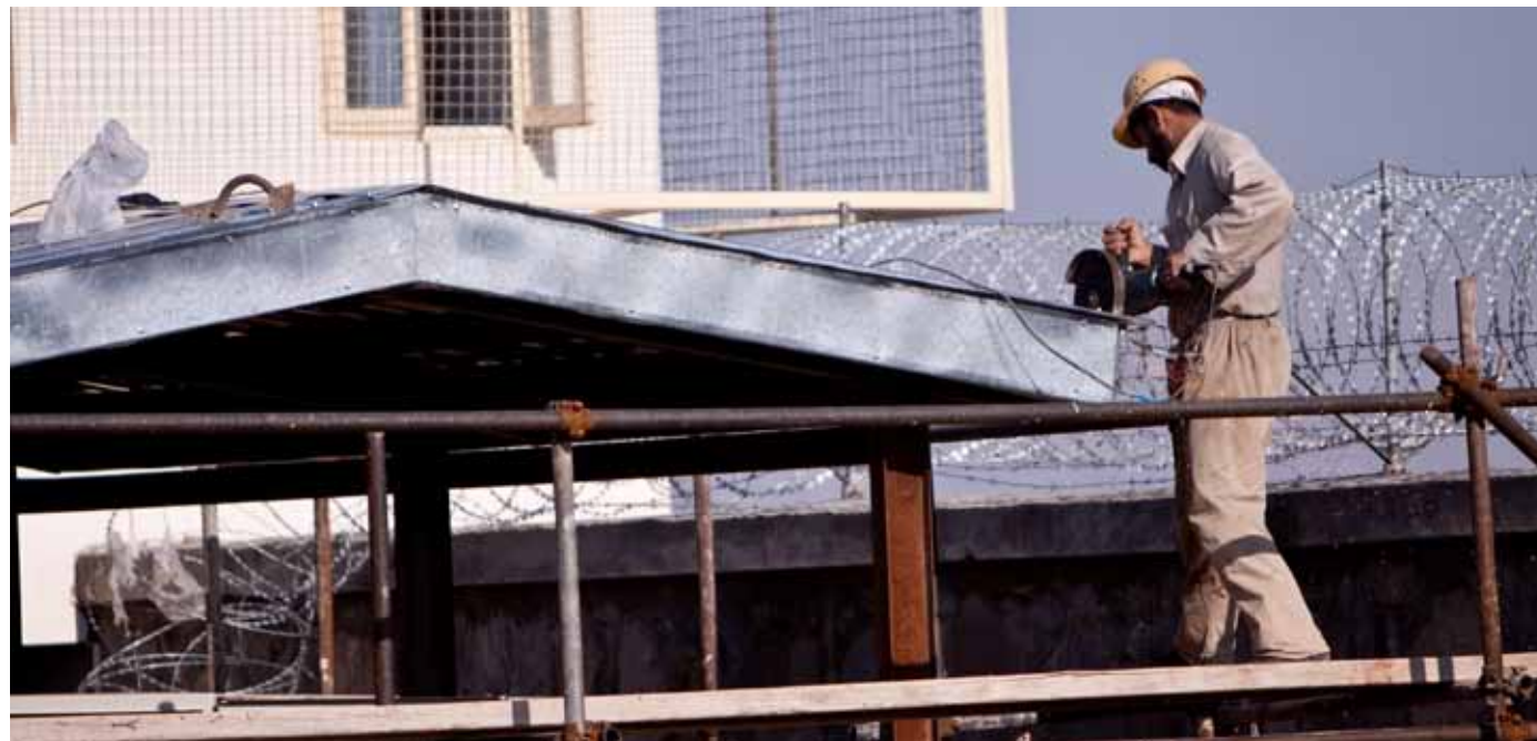
Afghan worker putting the finishing touches on the roof which will house a power generator for ANA compound. (Photo by Joe Marek)
