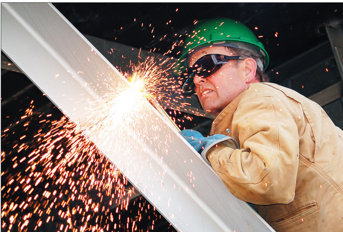
ABOVE: C a m Odekirk, 611th Civil Engineer Squadron mechanic, uses a cutting torch to remove support beams under the antenna prior to demolition. LEFT: The last antenna at the former Bethel Radio Relay Station is toppled to ease in its dismantling. The White Alice Communication System provided communications to remote parts of Alaska before modern telecommunications. (U.S. Air Force photo/Tommie Baker)
