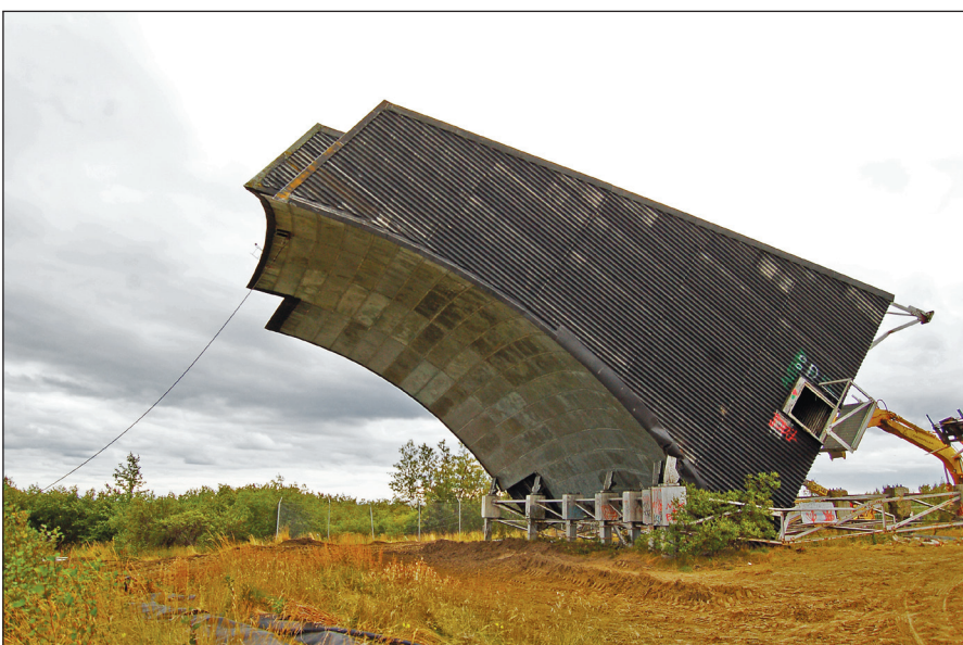
ABOVE: C a m Odekirk, 611th Civil Engineer Squadron mechanic, uses a cutting torch to remove support beams under the antenna prior to demolition. LEFT: The last antenna at the former Bethel Radio Relay Station is toppled to ease in its dismantling. The White Alice Communication System provided communications to remote parts of Alaska before modern telecommunications. (U.S. Air Force photo/Tommie Baker)
