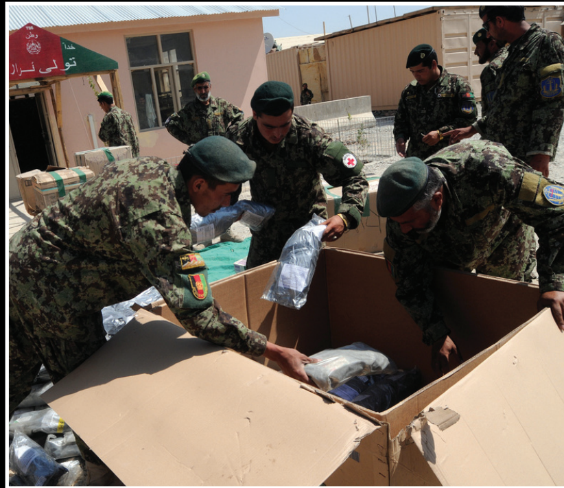
Afghan National Army soldiers unpack supplies as part of a Czech Provincial Reconstruction Team renovation of a dining hall and first aid station at Alitmur Base, Pul-e Alam District July 20. (Photo by Filip Moravec Czech Provincial Reconstruction Team)
