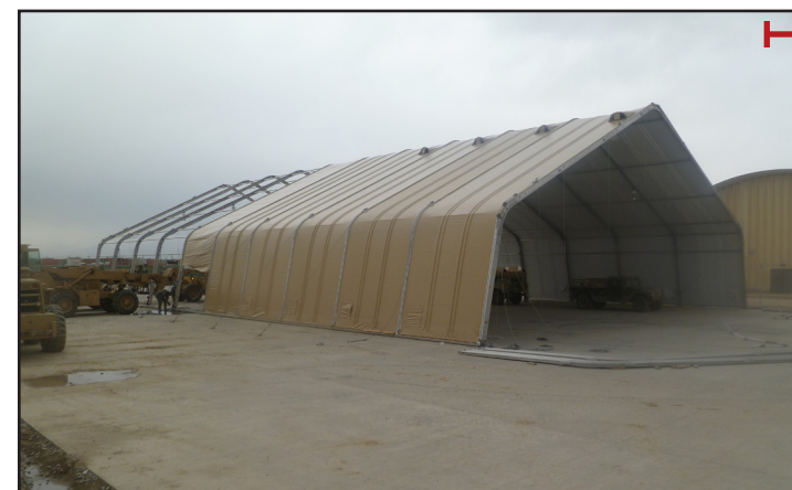
BAGRAM AIRFIELD, Afghanistan – Soldiers of Headquarters Support Company, Task Force Mountain Eagle, are constructing a Large Area Maintenance Shelter which will be used by the TF Mountain Eagle motor pool upon completion. (Photo by Sgt. George Tucker, TF Mountain Eagle, 10th Combat Aviation Brigade, 10th Mountain Division)
