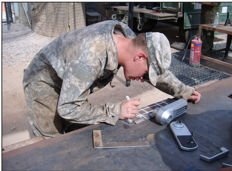
ABOVE—Sgt. Ricki French outlines where he will emplace a code-lock on a metal security door for the tactical operations center. ABOVE RIGHT—French tack-welds sections of metal together in the shop on COB Basra that will be used to create Silver Lion Battalion crest. NEXT PAGE—Members of Company F, 1st Bn., 68th Armor Reg., 3rd AAB, 4th Inf. Div., inspect sheet metal designs of the battalion crest.
