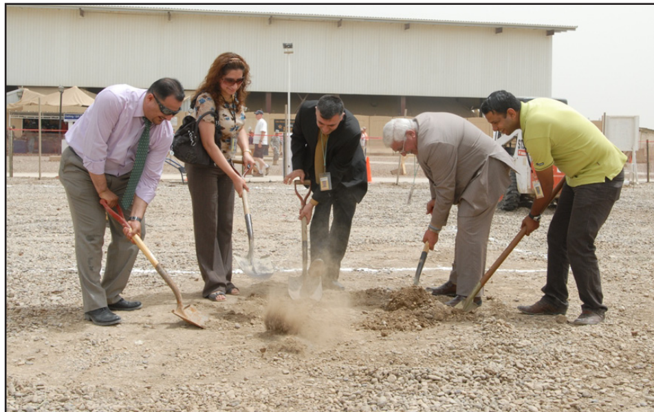
Bank of Baghdad employees break ground on Camp Liberty at the future home of the Bank of Baghdad. The Iraqi Based Industrial Zone’s Golden Construction Company is building the facility, which is scheduled to open in late July.
