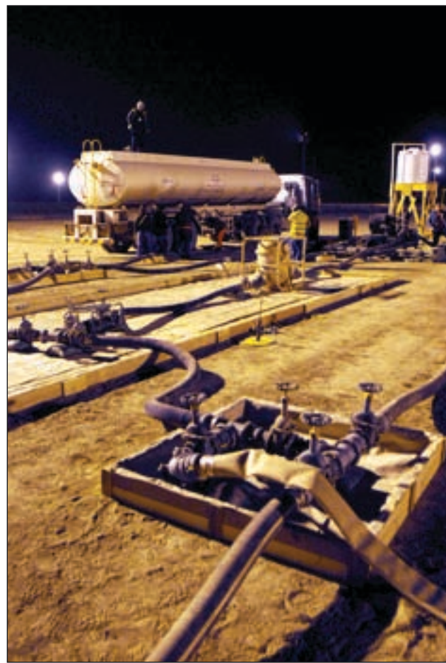
KBR, Inc. employees prepare to fill the first bag of motor gas Jan. 28 at the newly constructed fuel farm at Contingency Operating Base Adder, Iraq.
