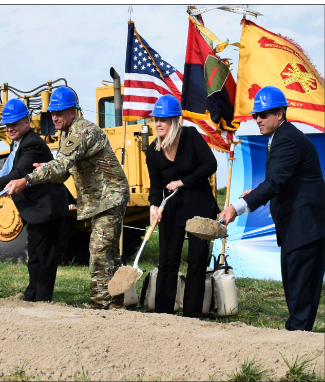
Corvias and Fort Riley leaders broke ground Oct. 1 in the Warner Peterson area construction site of 96 new homes. The homes are part of a series of housing projects already underway, an investment of $62 million in new construction, renovations and energy-efficient upgrades at Fort Riley. Pictured, from left to right: Steve Milton, chief, Housing Division, Fort Riley Public Works; Paige Callaway, Fort Riley resident and spouse of First Sgt. Cody Callaway, 1st Attack Reconnaissance Battalion, 1st Aviation Regiment, 1st Combat Aviation Brigade, 1st Infantry Division; Heath Burleson, partnership advisor, Corvias; Col. Stephen Shrader, U.S. Army Garrison Fort Riley commander; Angela Watson, operations director, Corvias-Fort Riley; Kelly Karl, director of construction, Corvias.
