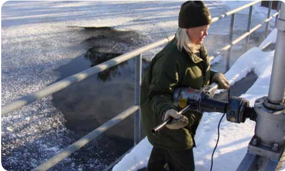
Mary Kay Larson, Gull Lake Recreation Area park manager, operates the dam during a gate change. Photo by Brian Turner
