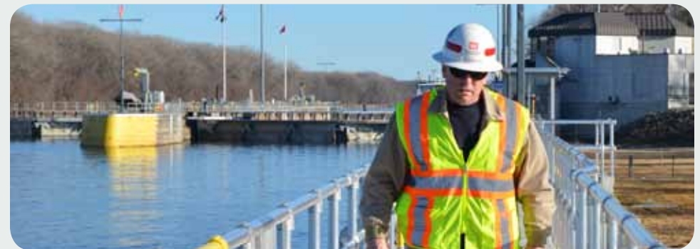
Eric Johnson, engineering and construction, monitors construction at Lock and Dam 3, near Red Wing, Minn., Jan. 10, 2012.
