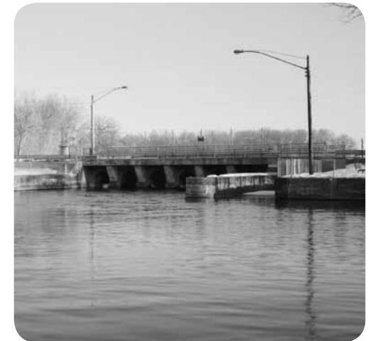
The Gull Lake Dam, near Brainerd, Minn., is the only one of the six Headwaters dams to be initially constructed in concrete. The dam was placed into operation 101 years ago in 1912. Photo by Patrick Moes
