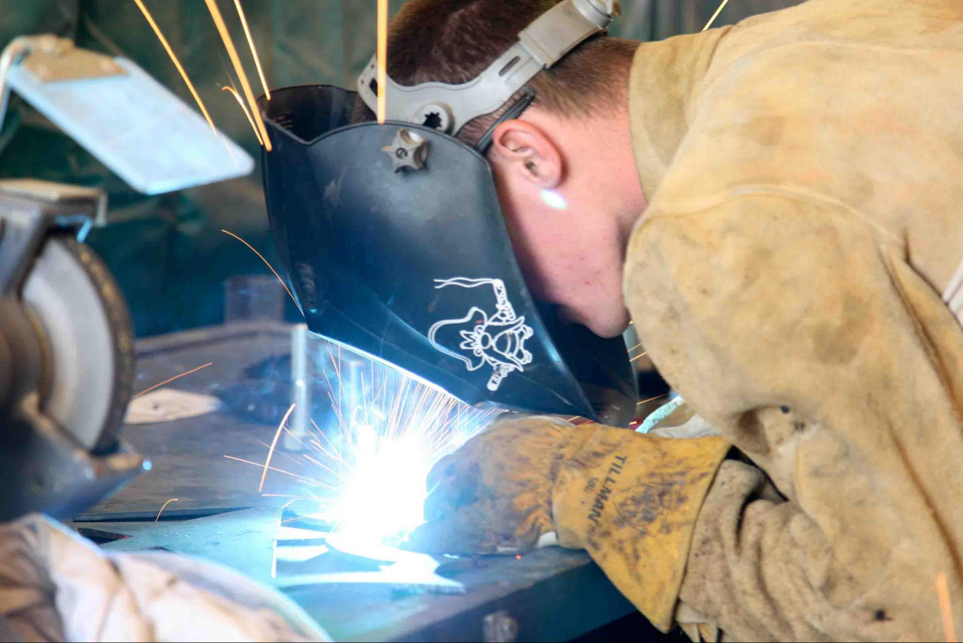
U.S. Army Pfc. Nicholas Dizenzo, a wheeled vehicle mechanic with Fox Company, 3rd Battalion (Airborne), 509th Infantry Regiment, Task Force 4-25, welds a bolt to a custom shelf bracket on Forward Operating Base Gardez, Paktia province, Afghanistan, Aug. 25, 2012. (U.S. Army photo by Sgt. Kimberly Trumbull / Released)
