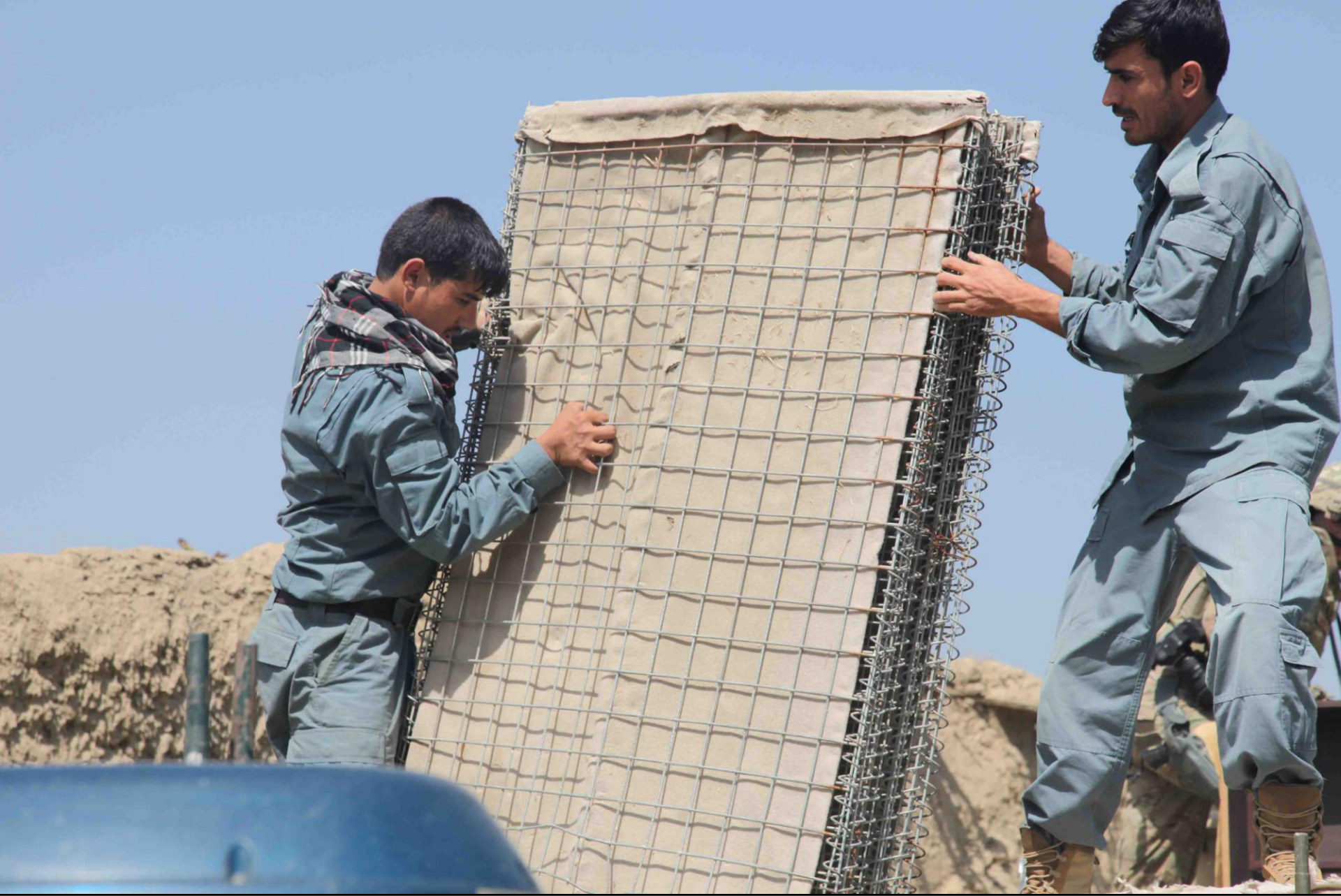
Afghan National Police (ANP) officers unload a Hesco barrier off a truck outside of an ANP compound in Parwan province, Afghanistan, Sept. 22, 2012. The ANP are going to use the barriers to better secure their compound. (U.S. Army photo by Spc. Andrew Claire Baker/Released)
