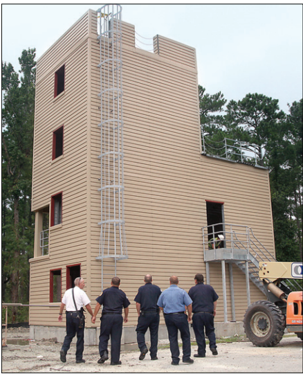
Cherry Point Fire and Emergency Services firefighters survey the progress of their new training tower here Aug. 24. The new training tower has two additional stories and up-to-date equipment inside to help the firefighters train.
