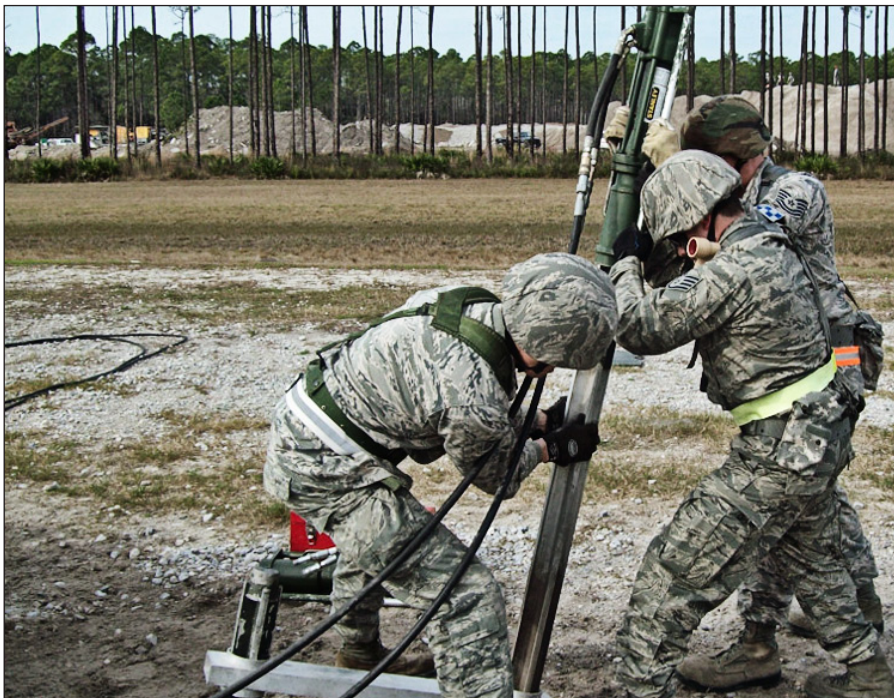
124th Civil Engineer Squadron power production specialists construct a mobile aircraft arresting system during their weeklong Silver Flag exercise in February at Tyndall Air Force Base, Fla. (Photo courtesy of 124 CES)
