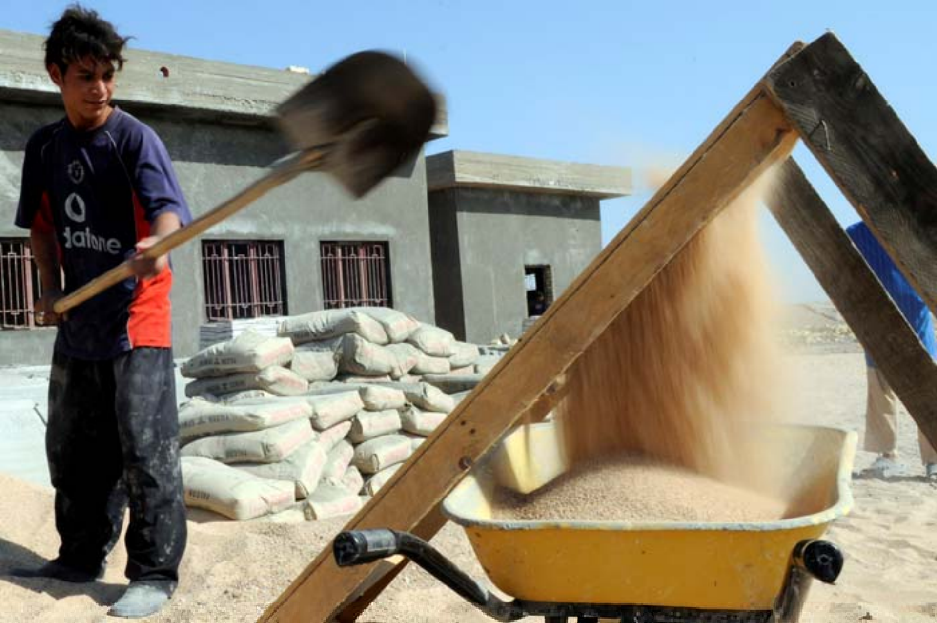
A young boy uses a sieve to sift through the sand to remove coarse materials as U.S. Soldiers from the 1314th Civil Affairs Company, 17th Fires Brigade, and Iraqi soldiers, conduct a foot patrol to the Al Mayah and Rota Schools, to carry out the project purchasing officer's final Commander Emergency Response Program (CERP) assessments, in Basra, Iraq, Oct. 21, 2009. (U.S. Air Force photo by Staff Sgt. Chrissy Best/Released) 091021-F-2575B-095
