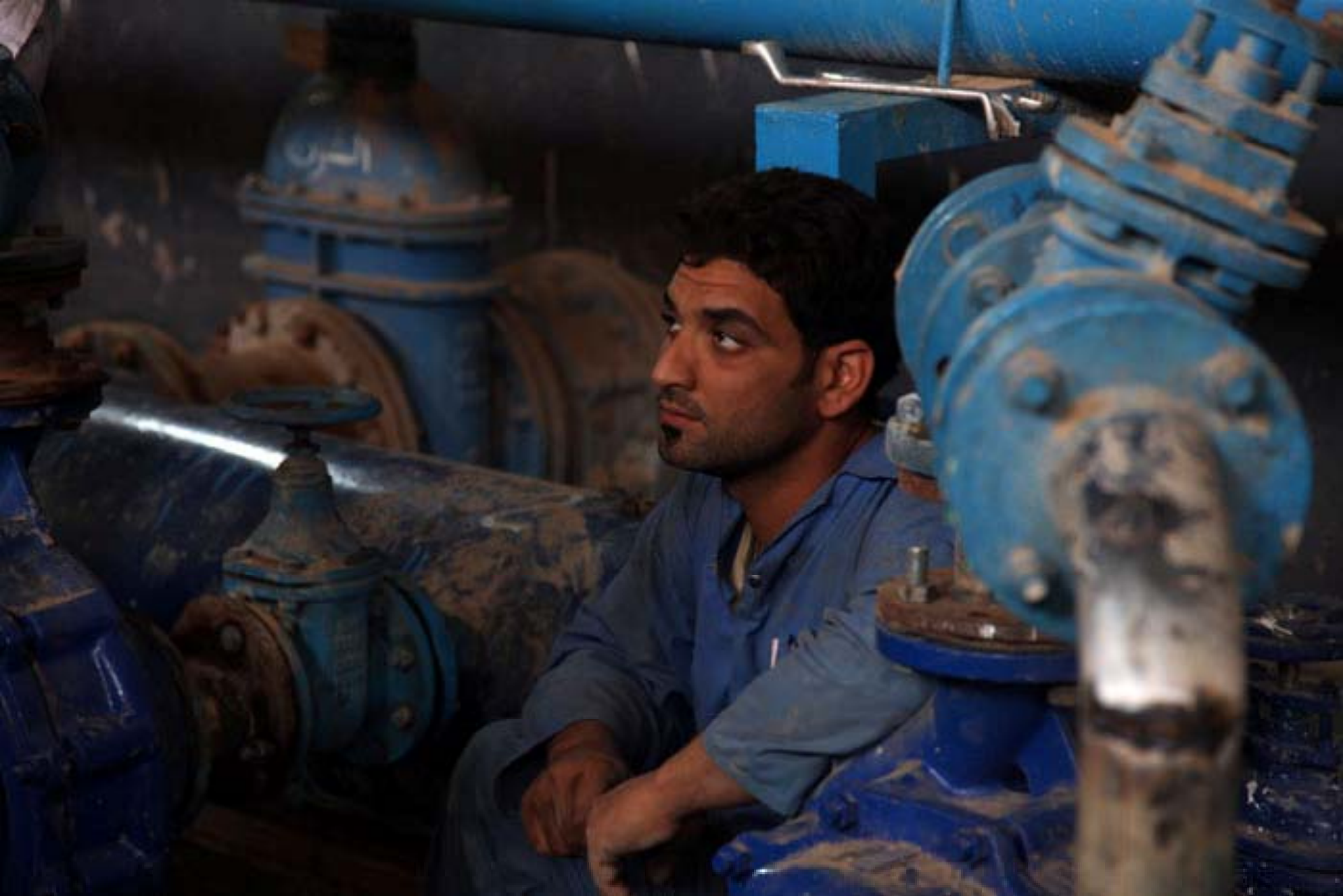
A worker listens as members of the Al Anbar Provincial Reconstruction Team (PRT) discuss improvements for a water treatment plant in Hadamiyah, Iraq, Oct.29, 2009. The Al Anbar PRT conducted a project assessment of the water treatment and power plants in the area.
