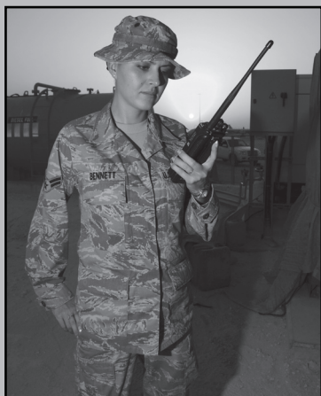
Airman 1st Class Christina Bennett, 379th Expeditionary Civil Engineer Squadron force protection and security escort, maintains accountability of Third Country National workers at the Base Defense Operations Center construction site, Sept. 29. (U.S. Air Force photo/Tech. Sgt. Jason Edwards)
